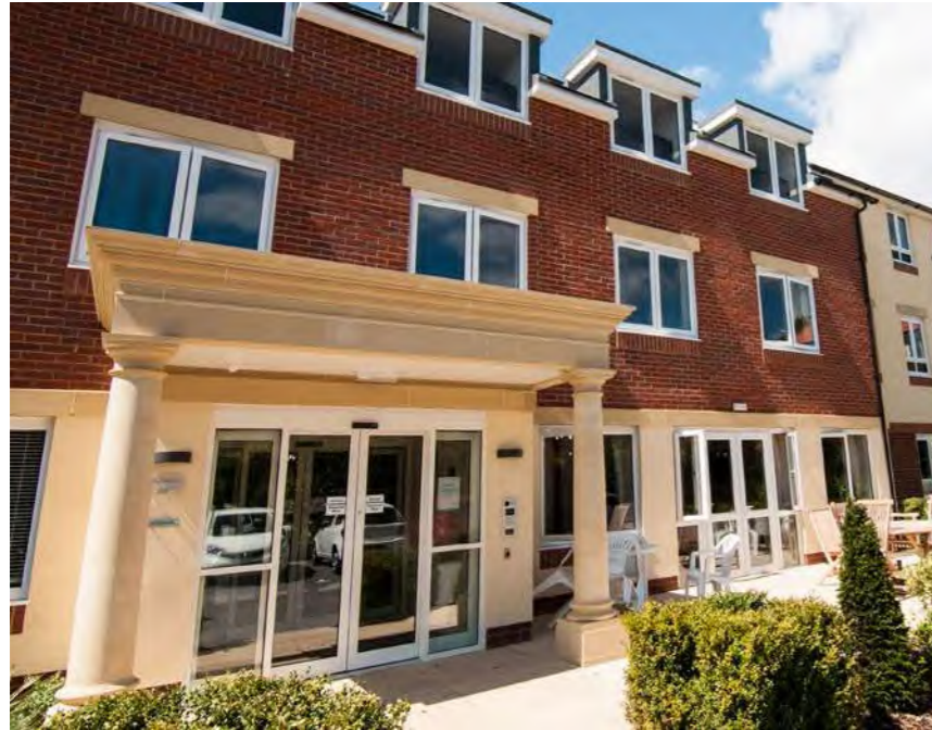
Secure Main Entrance from Parking
